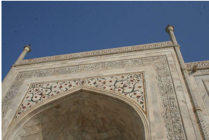
Fig. 13 South facing facade from the plinth
