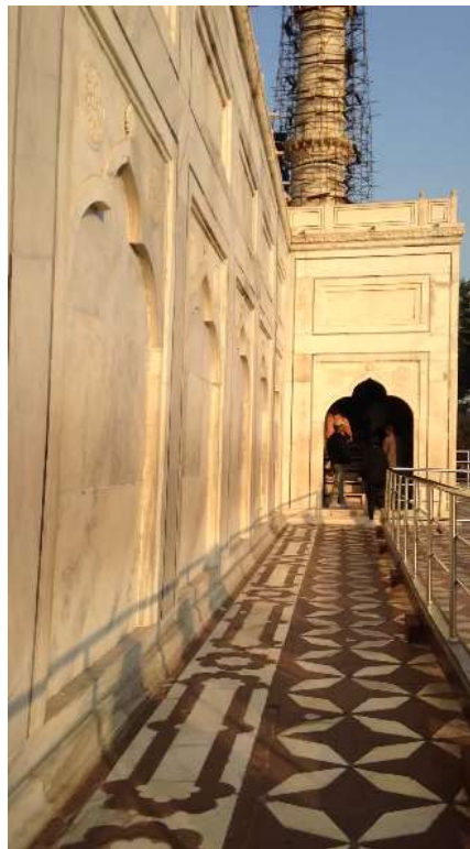
Fig. 12 Stairs onto the Plinth looking east
