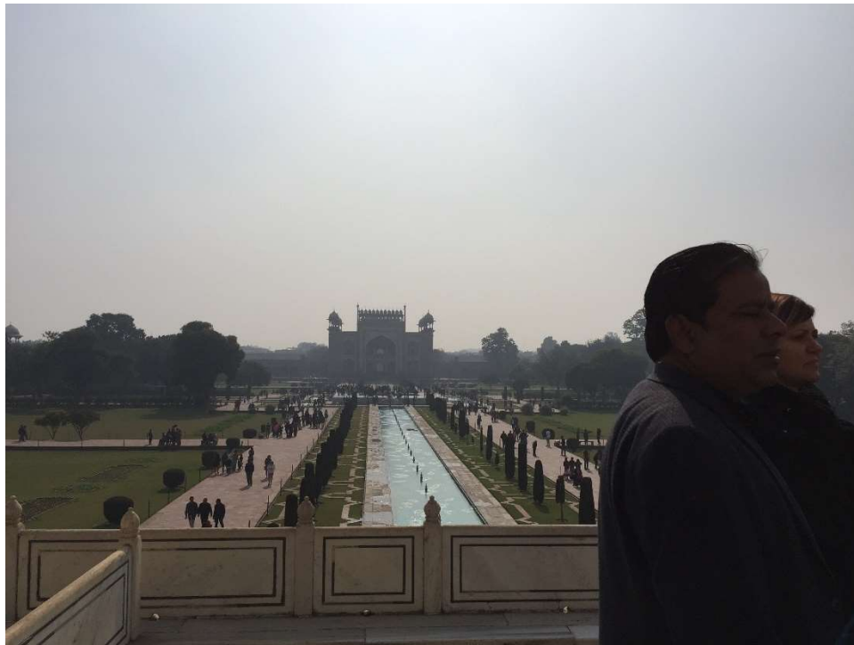
Fig. 31 Gardens from the plinth looking south
